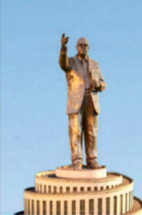
BHARAT RATNA DR. BHIM RAO AMBEDKAR INDIA MILE, DADAR, MAHARASHTRA TOTAL HEIGHT 490 FEET (151 METERS) STATUE HEIGHT 350 FEET (106.68 METERS) WORK IN PROGRESS
